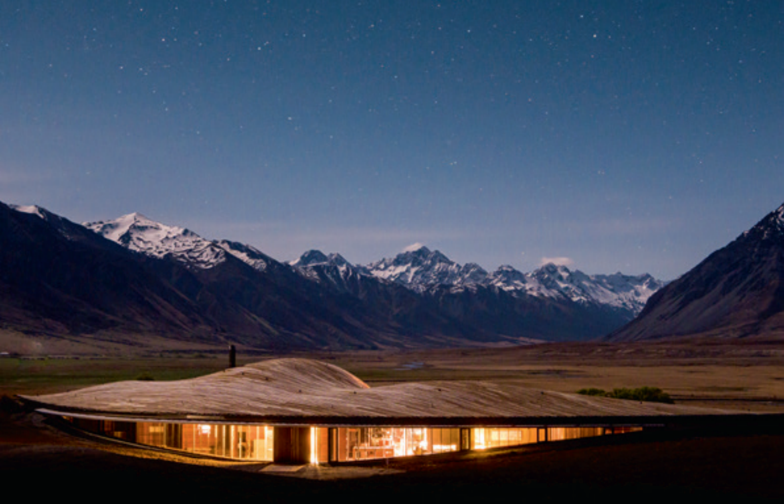
The sweeping, curved roofline of The Lindis blends seamlessly into the majestic terrain of South Island's remote Ahuriri Valley.
